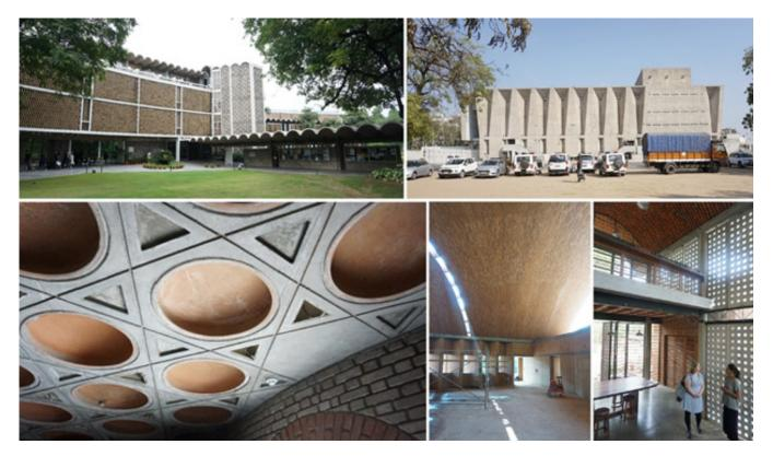
Figure 1. Clockwise from top-left a) The India International Center by J. A. Stein and Binoy Chatterjee, New Delhi, 1962 b) Tagore Memorial Hall by BV Doshi and Mahendra Raj, Ahmedabad, 1965 c) Ferrocement panels, vaulted roof, and filler slab in Wall House by by Anupama Kundoo, Auroville, 2000 c) Long-spanning masonry and concrete vault at Auroville Earth Institute e) Filler slab; Development Alternatives Headquarters by Ashok B. Lall Architects, New Delhi, 2014.
